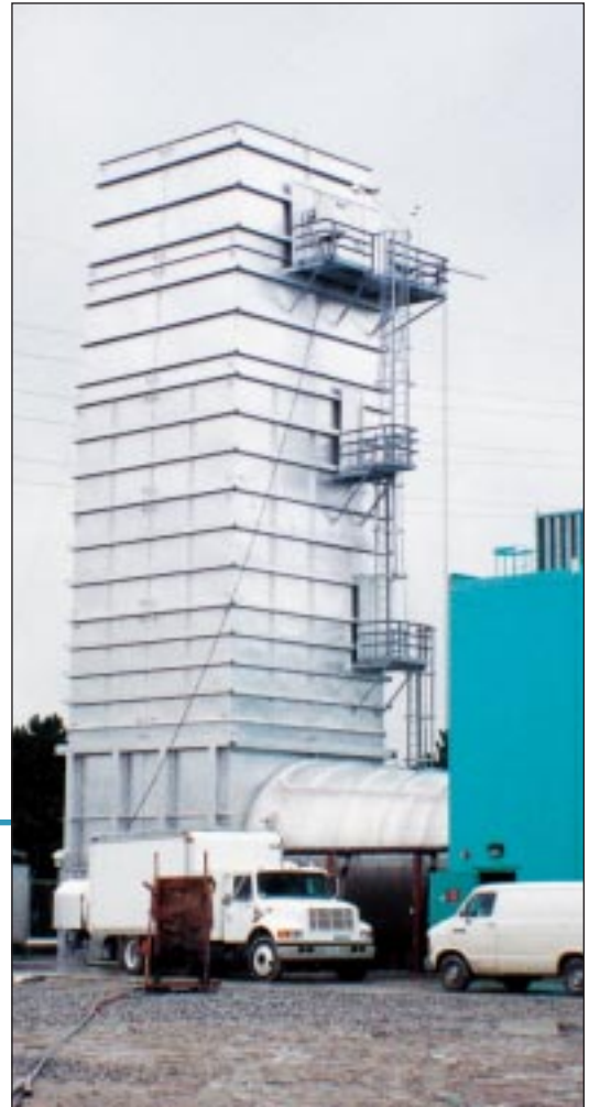
75' tall system for a V84.2, designed for a low-noise site.
