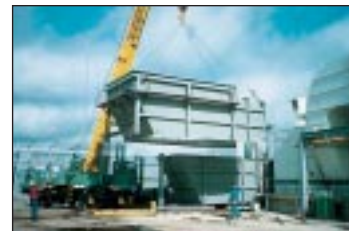
Assembly of rectangular exhaust stack.
