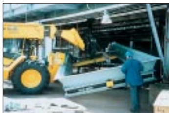
Installation of Braden B-Flex expansion joint.
