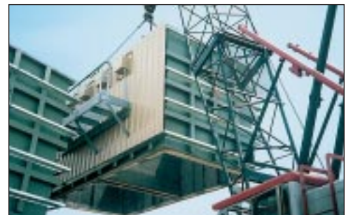
Installation of preassembled upper stack section showing platforms, lagging, and instrumentation.
