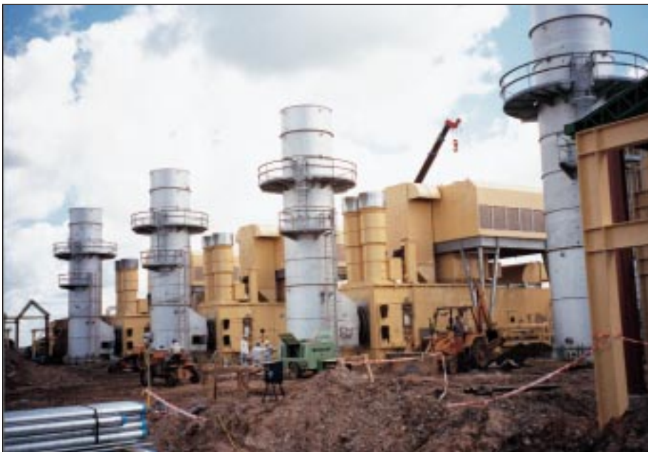
50' tall LM6000 exhaust system, Guyaquil, Ecuador.
