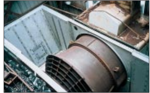
Exhaust plenum installation.
