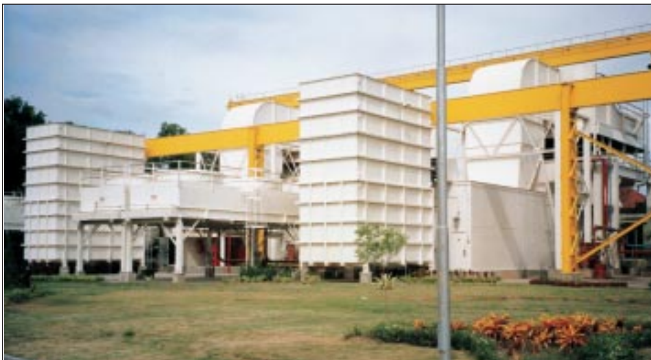
30' tall rectangular exhaust for two W251 units in Bali, Indonesia.
